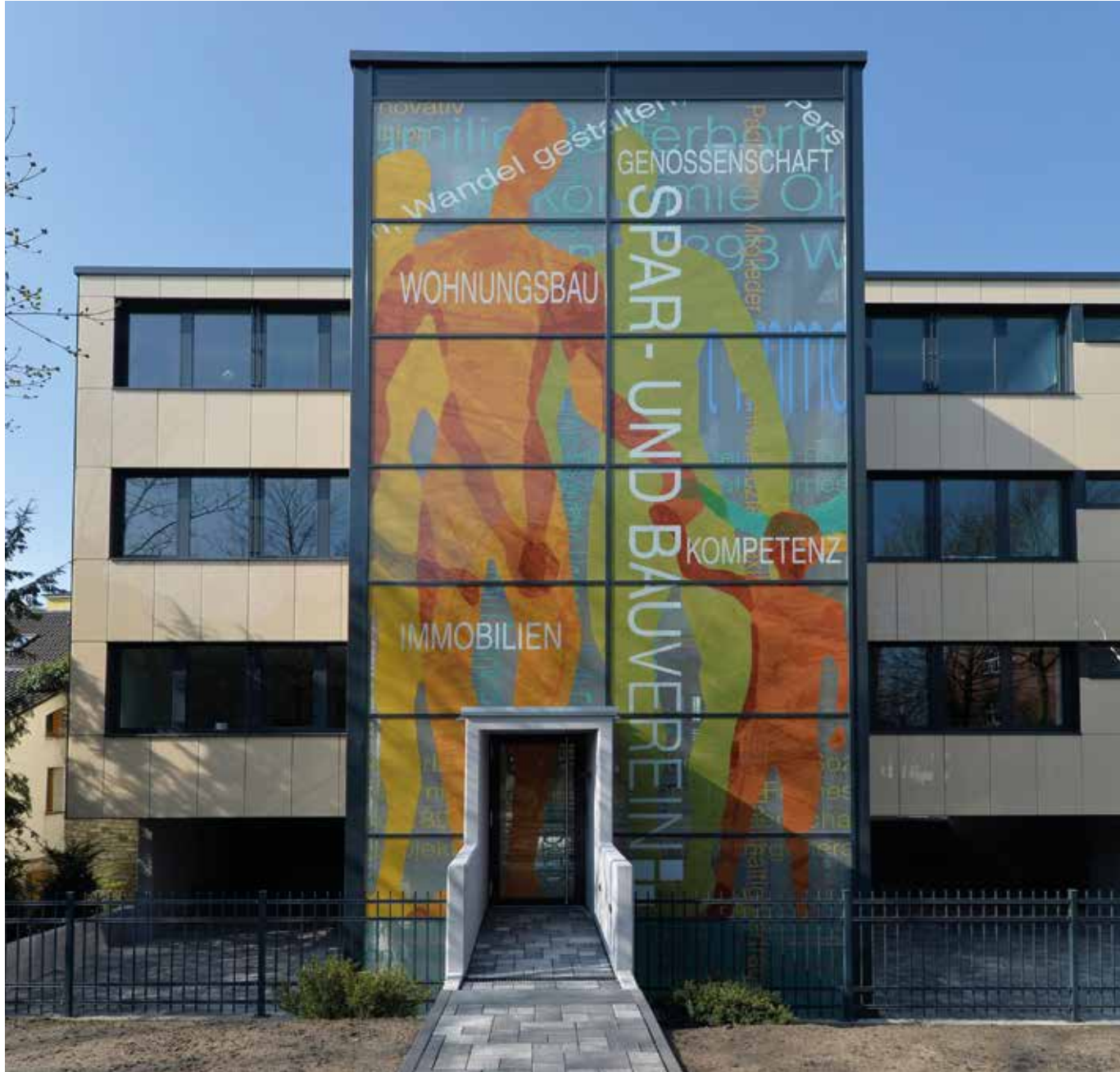
Company building of the Spar- und Bauverein, Paderborn, Germany – Artist: Martin Donlin
